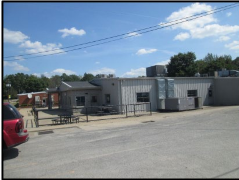
BUILDING 1412 – DINING HALL
