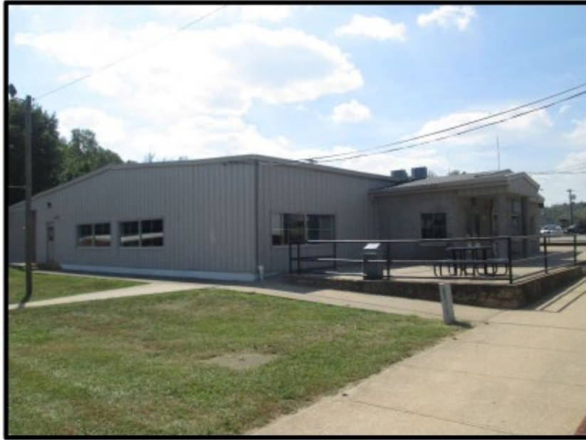
BUILDING 1412 - DINING HALL
